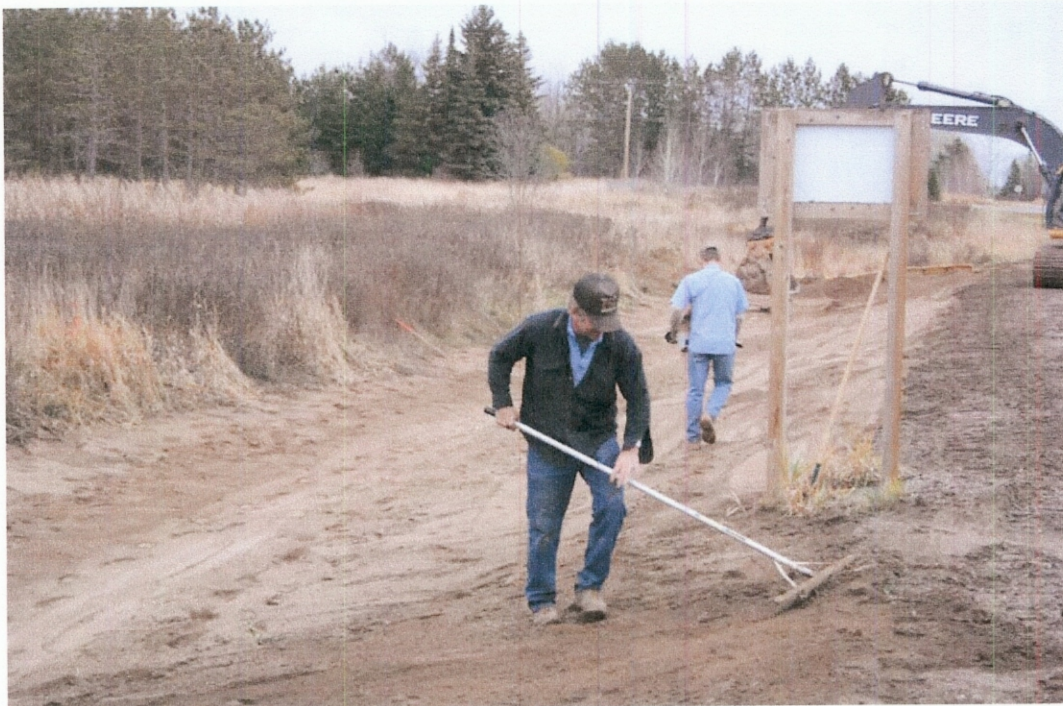
Photograph 6. Placement of topsoil was completed on November 7, 2008. Hand rotary seeding and raking in of seed was completed as well on November 7, 2008. Photo taken facing east.
